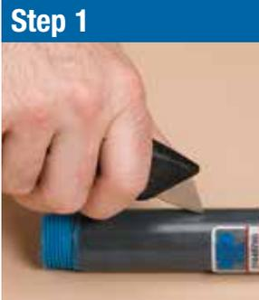
**Step 1** consists of two cuts through the plastic to the substrate along the length of the conduit at approximately 1/2" apart, three to four inches in length. A third perpendicular cut crosses the lengthwise cuts.
